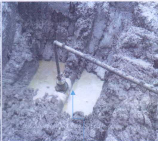
AFTER EXCAVATION (SPILL POINT)
